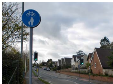
Picture 9 Signal controlled crossing at Monks Lane
